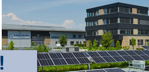
New office in Oberessendorf
